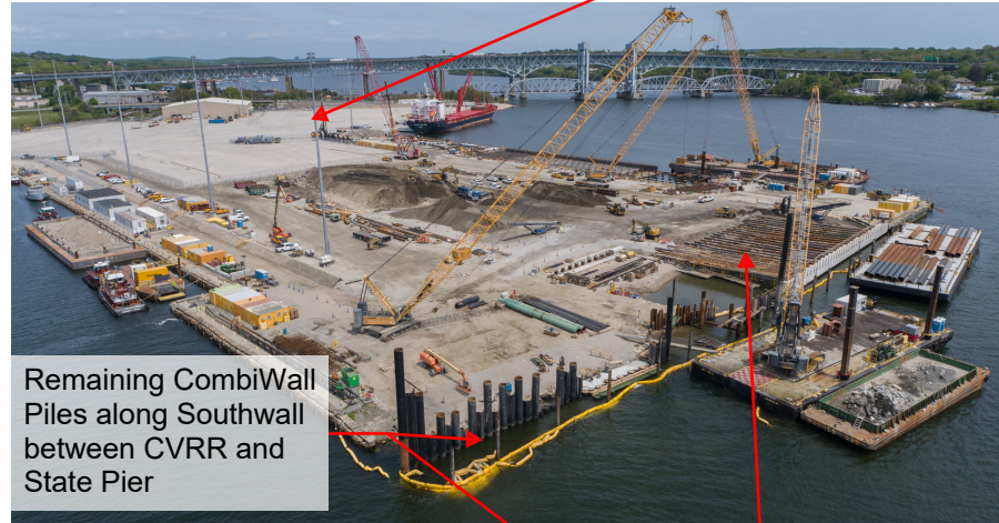
High Mast Lighting
