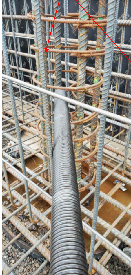
Delivery Berth Combi-wall cap reinforcement
