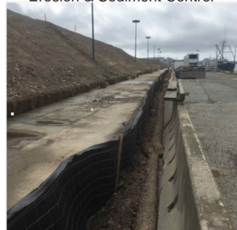
Stock Pile of Fill Material for the Central Wharf In-fill Operation
