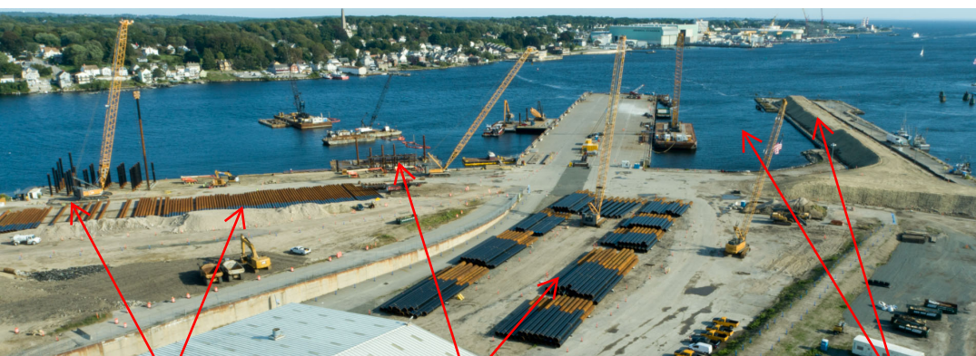
Delivery Berth & Heavy Lift Platform 30 inch Steel Pipe Pile
