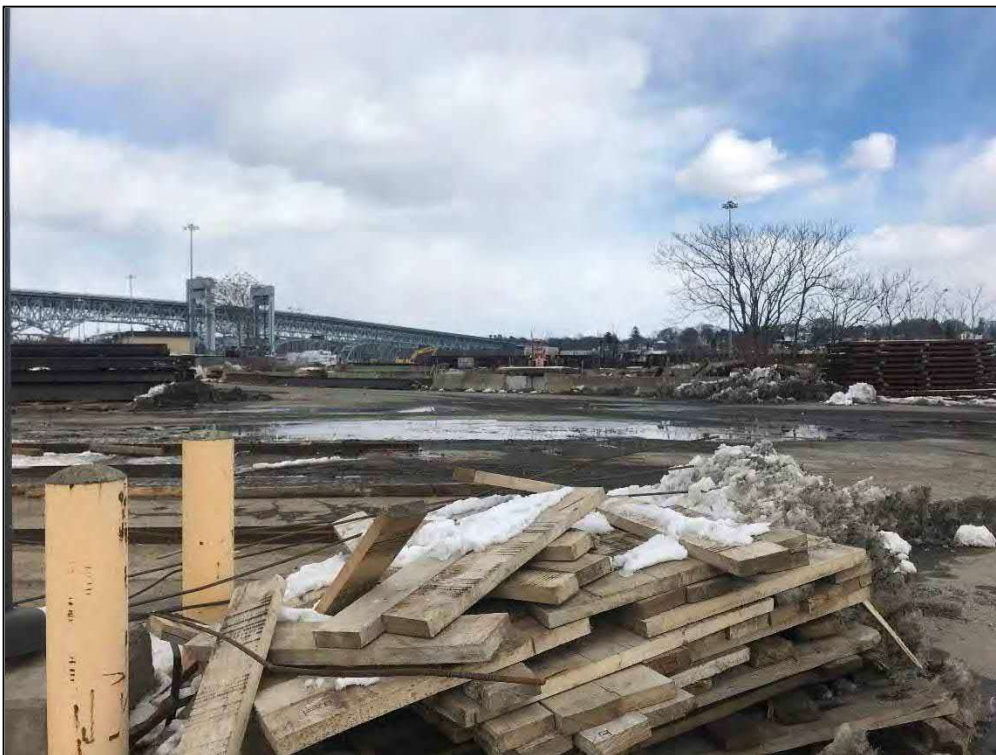
14. View northeast of the shoreline section adjacent to the pier from the top of the pier, looking toward the Gold Star Memorial Bridge.
