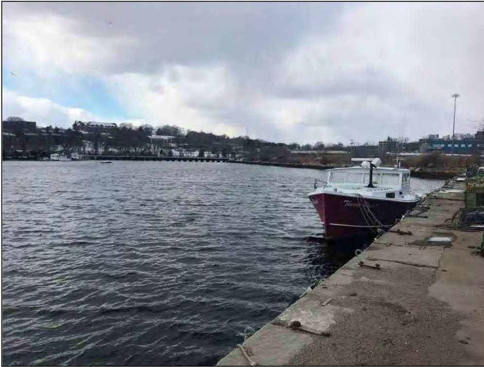
11. View northwest from west side of pier, looking toward New London.
