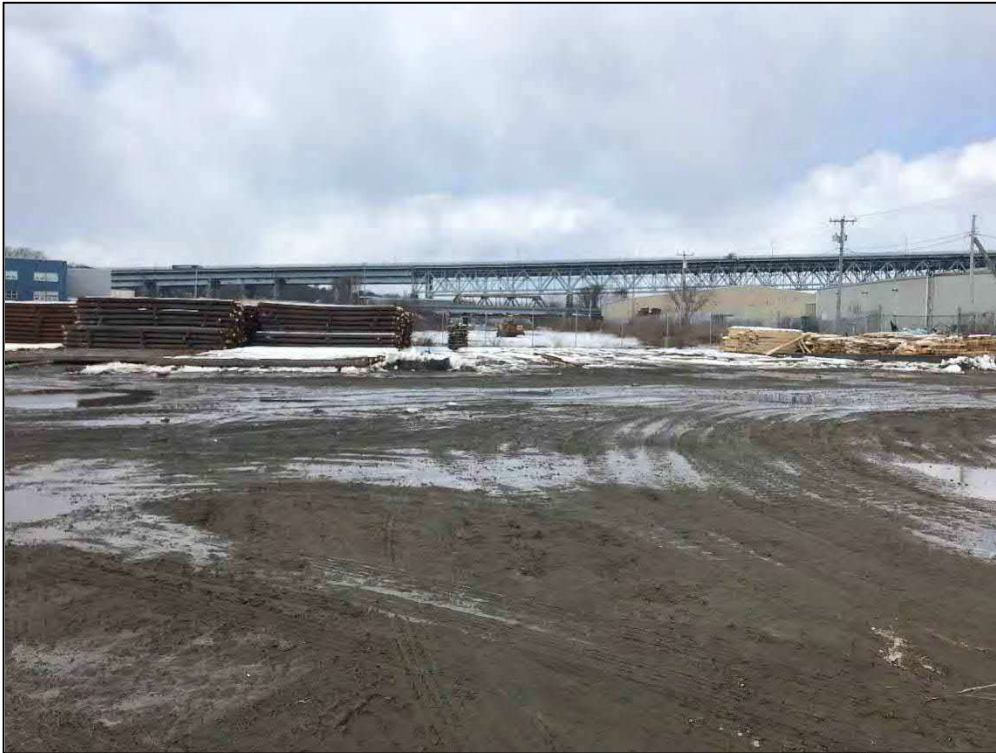
13. View north of the shoreline section adjacent to the pier from the top of the pier, with the Gold Star Memorial Bridge in the background.
