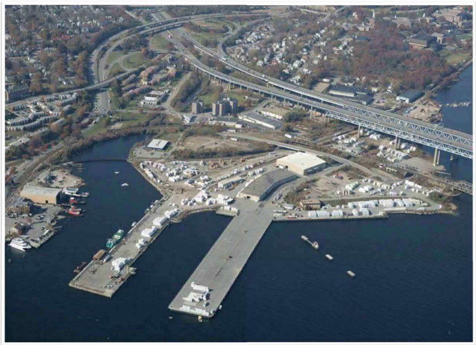
FIGURE 1: EXISTING SITE OVERVIEW OF THE STATE PIER
