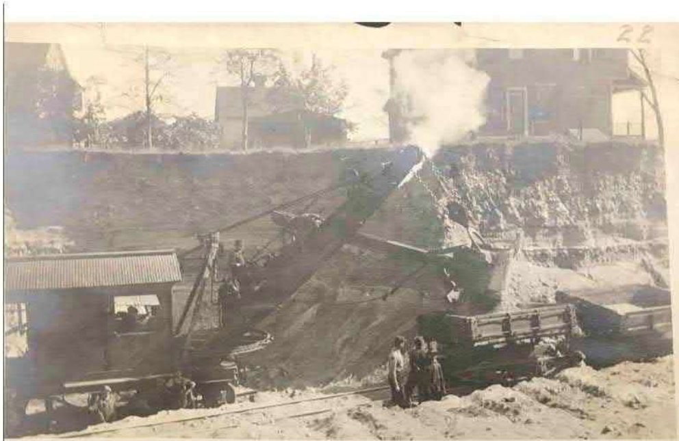
Photograph 3: View of bluff cut to accommodate the rail spur. Note stratigraphy, indicating multiple depositional events at depth (yellow arrows). Facing east. Courtesy of the New London County Historical Society Archives.
