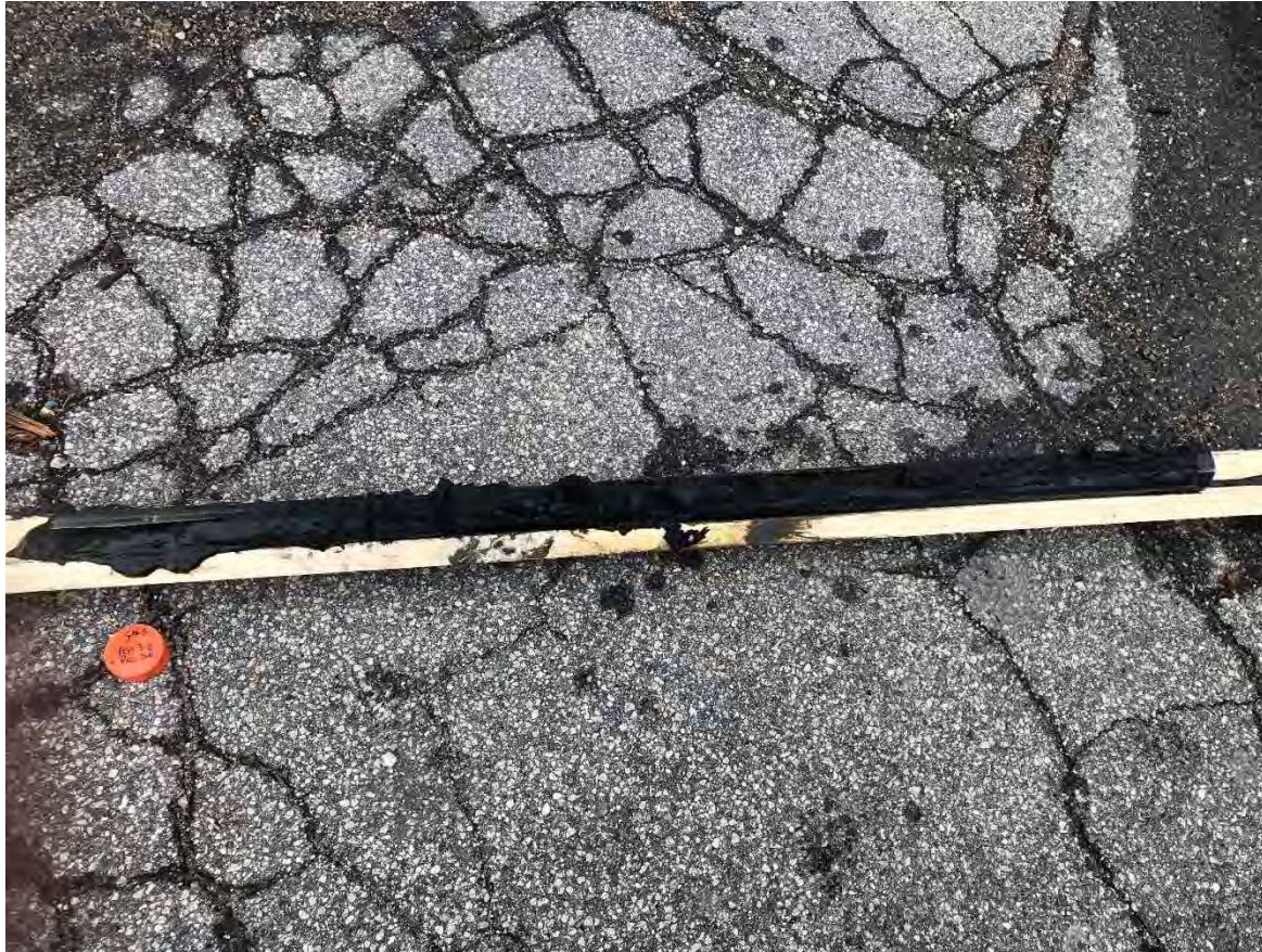
Photo 1: View of Chem-5. Run from left to right, 0 to 3.8 ft.
