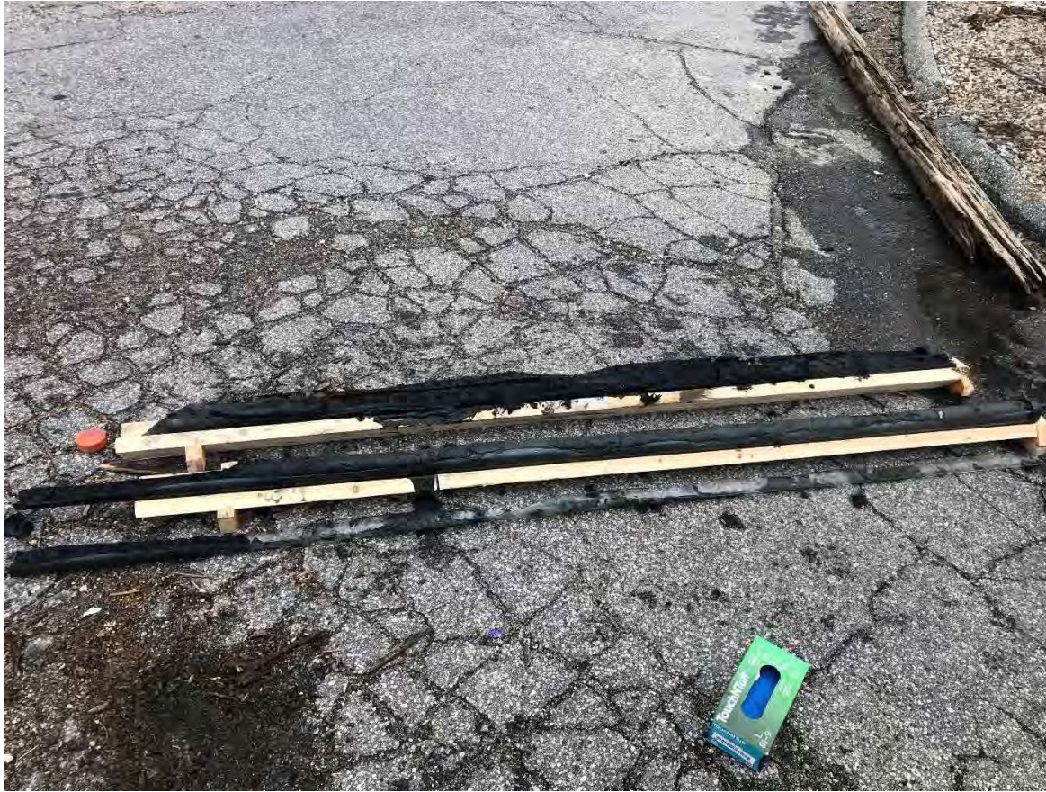
Photo 1: View of Chem-9. Top run from left to right from 0 to 12.6 ft, bottom run from left to right 12.6 ft to 21.8 ft.
