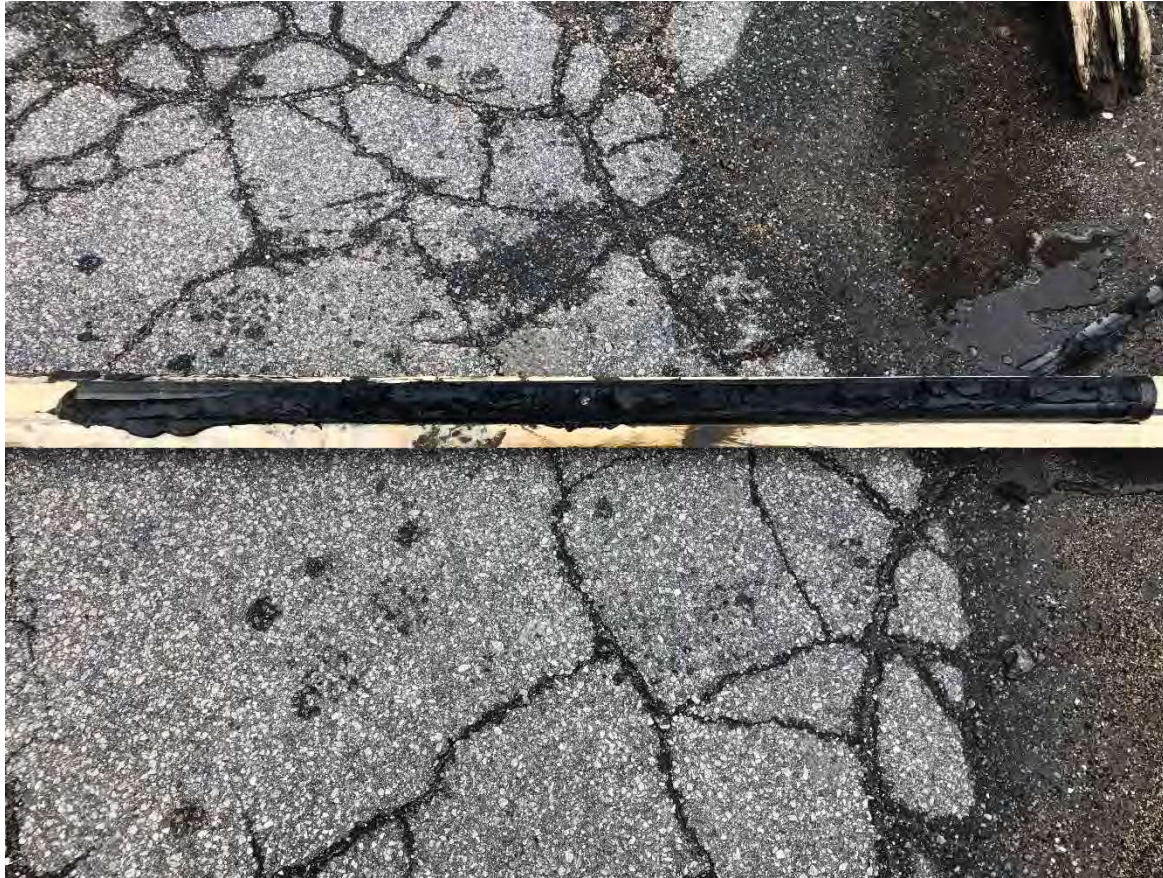
Photo 1: View of Chem-3. Run from left to right, 0 to 3.5 ft.
